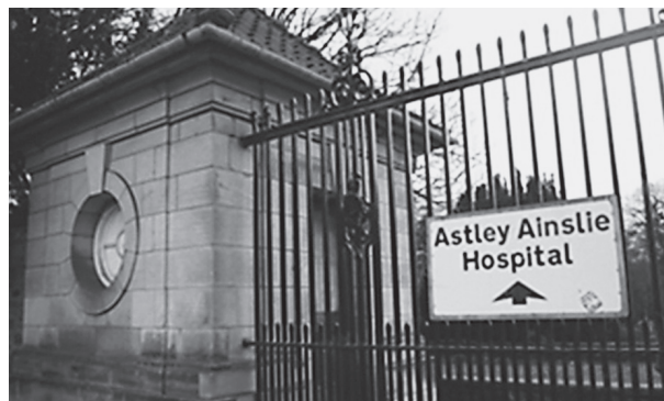
図3 Astley Ainslie Center 玄関
